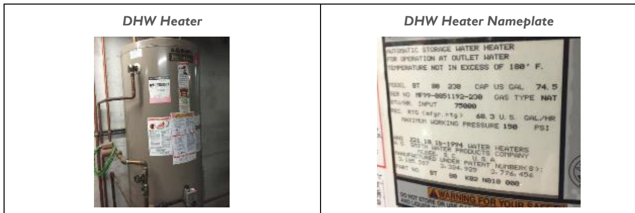
Figure 12 – Domestic Hot Water System
